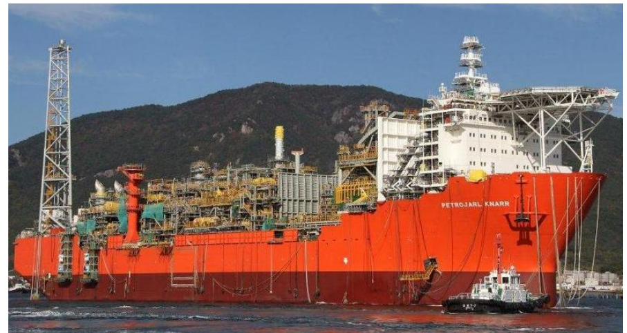
Top Side Installation (Jan-2014)
